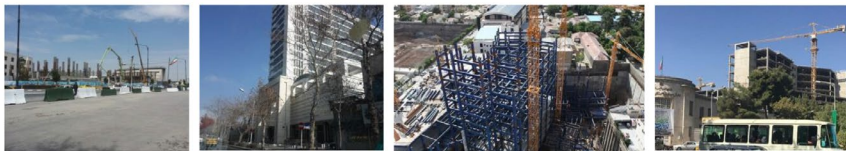
Figure 6. Mega-scale buildings. Source: the authors' field observation and official documents
