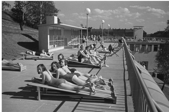
Fig. 18–19 Vanadisbadet, with children playing in the water streams at the end of the pool. Behind the pool; part of the modern funkis building with a café inside and an area for sunbathing on the roof. Vanadisbadet, Stockholm, 17 May 1938. Photos: Gunnar Lundh (GL.129072, GL.129085).
