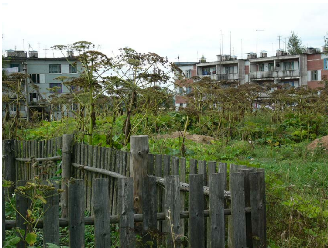
Figure 3 Block houses at the centre of Lavry. 2004. Photo: Aija Lulle
