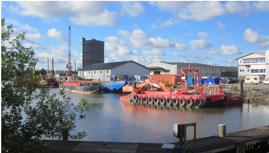
While walking past the well-established company Frog Marine Services, all the random visitor sees is a closed-off warehouse, an old barge moored in one of the harbour basins, and a couple of dredgers standing in the water. Photo: by the author.
